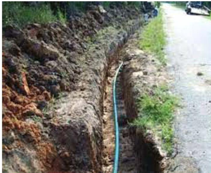
Modern Sewer Trench
