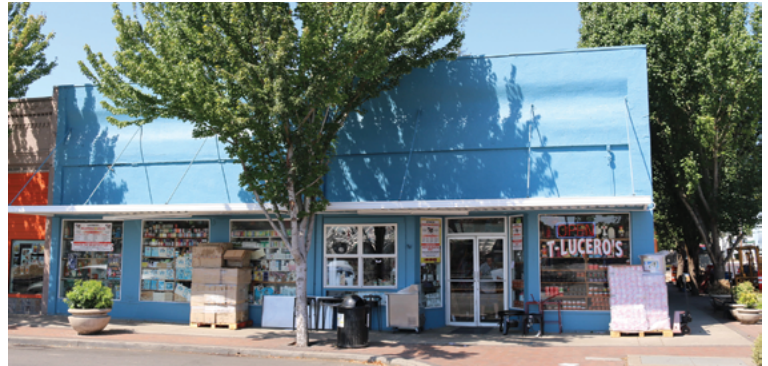
Before (top) and after facade improvements
