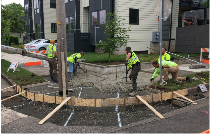
Workers at one of the Portland test sites moving wet concrete.
