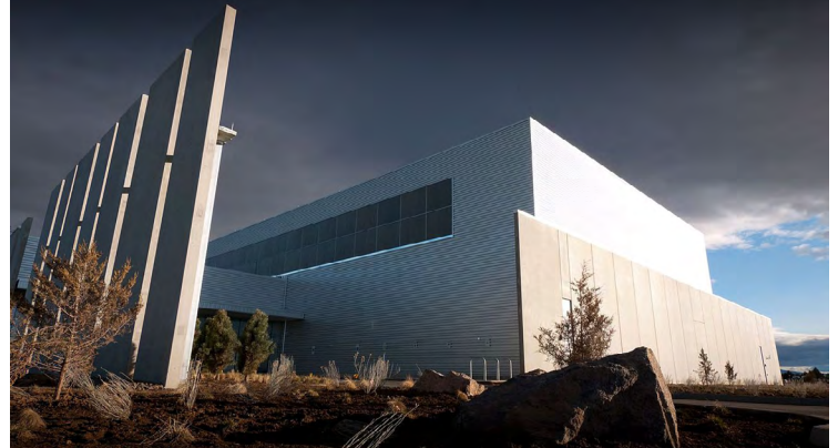
Facebook Data Center in Prineville
