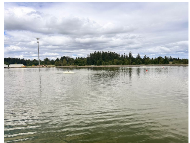
Lagoons at the city's wastewater treatment facility
