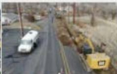
Geer Road Water Line Extension
