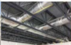
Treatment Plant Admin Building HVAC Upgrades
