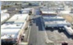
W. Hermiston Avenue Overlay
