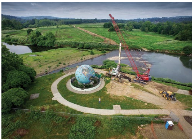
The Peter Courtney Minto Island Bridge construction site
