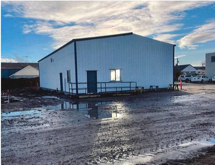
Nyssa's public works building project will include a new shop and lean-to, all enclosed by fencing
